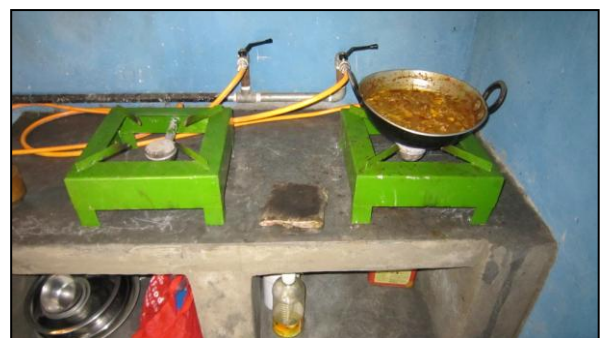
Fig.10:- The stove burns and food is cooked using the gas produced by the system.
