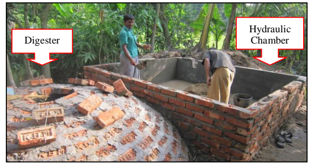
Fig. 7:- The construction of outer structure of the digester and hydraulic chamber
