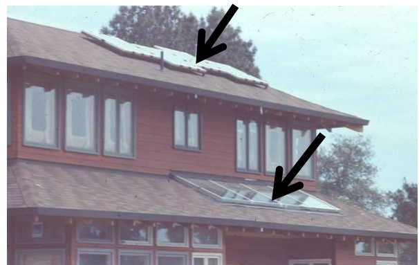
Fig. 5: Photovoltaic electricity generation and integrated passive solar hot water heating.
