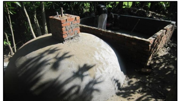
Fig. 9:- The complete structure of the digester and hydraulic chamber
