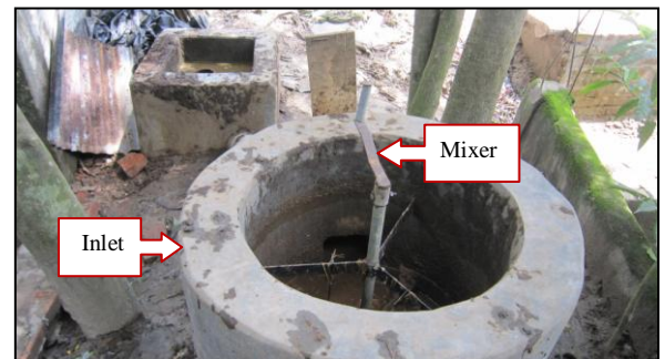
Fig. 8:- The Inlet of the system with mixer
