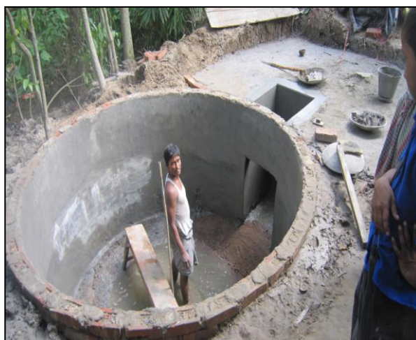
Fig. 6:- The base construction of the digester and hydraulic chamber
